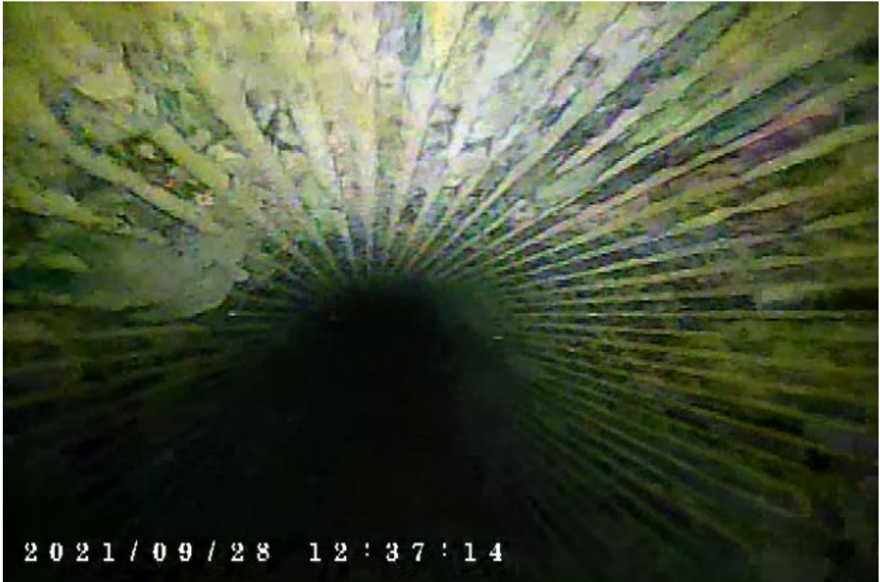
Figure A-2. Downhole image of the interior of Well 6. Well 6 had a substantial buildup in many sections of the well screen, so the well screen was rehabilitated.
